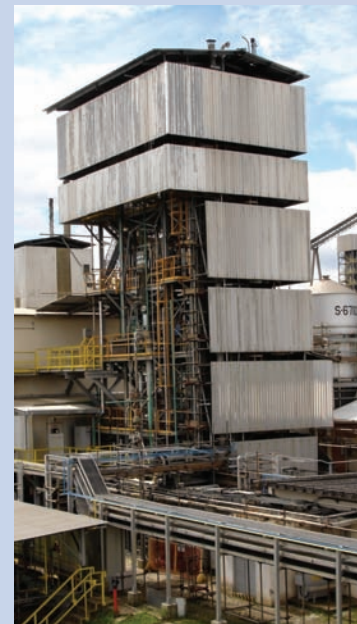
Fluid Catalytic Cracking unit - Oxy-firing demonstration, Brazil (image: Petrobras)
